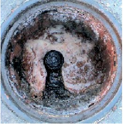
Prior to Treatment
